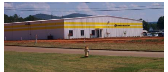
Changer & Dresser Corp.'s new facility off of Hillyer-Robinson Pkwy in Anniston.
